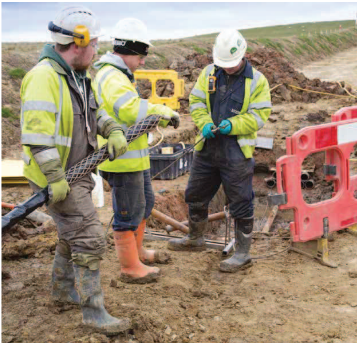
Cable pulling preparation
