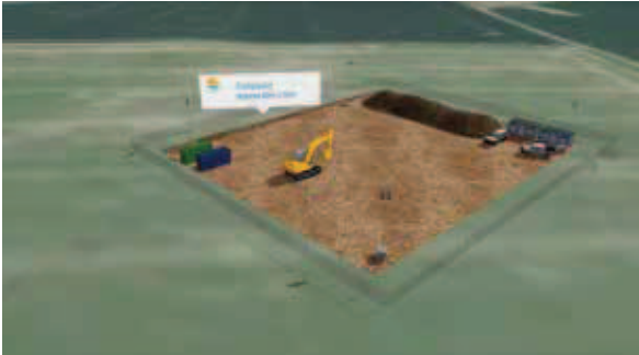
1. Site establishment including topsoil strip and store
