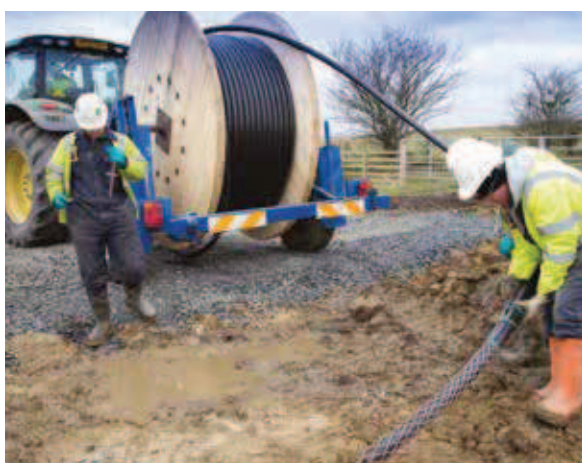
7. Pull cables into ducts
