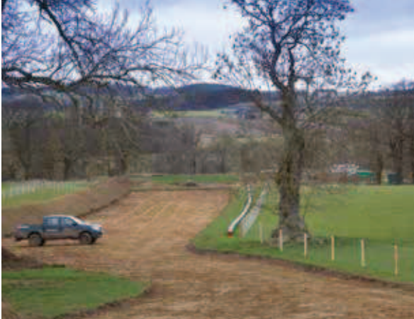
1. Topsoil Strip and Store
