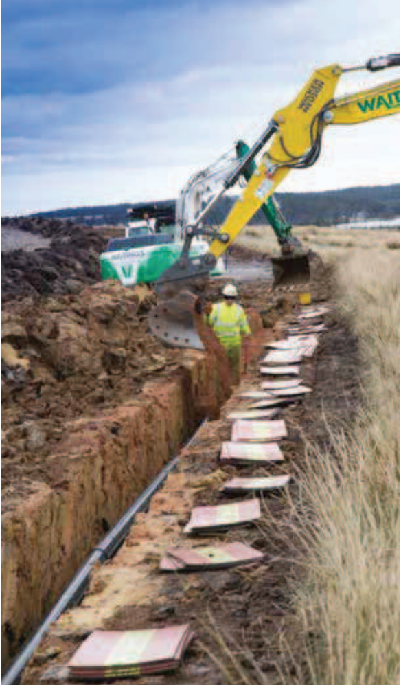
3. Ducts Covered and Protective Marker Tiles Laid
